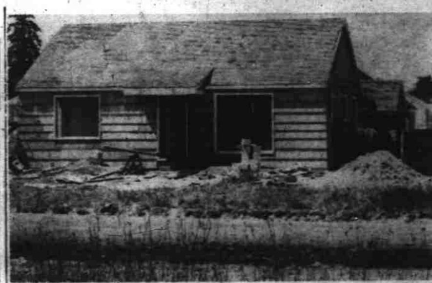
Lansing avenue are new homes of the type shown in the above picture being constructed by P. W. Harcourt, Salem contractor. Part of a large project, the house shown above will soon be finished. Other homes built by Harcourt on Lansing avenue are already occupied. (House photos by Don Dill, Statesman staff photographer.)
