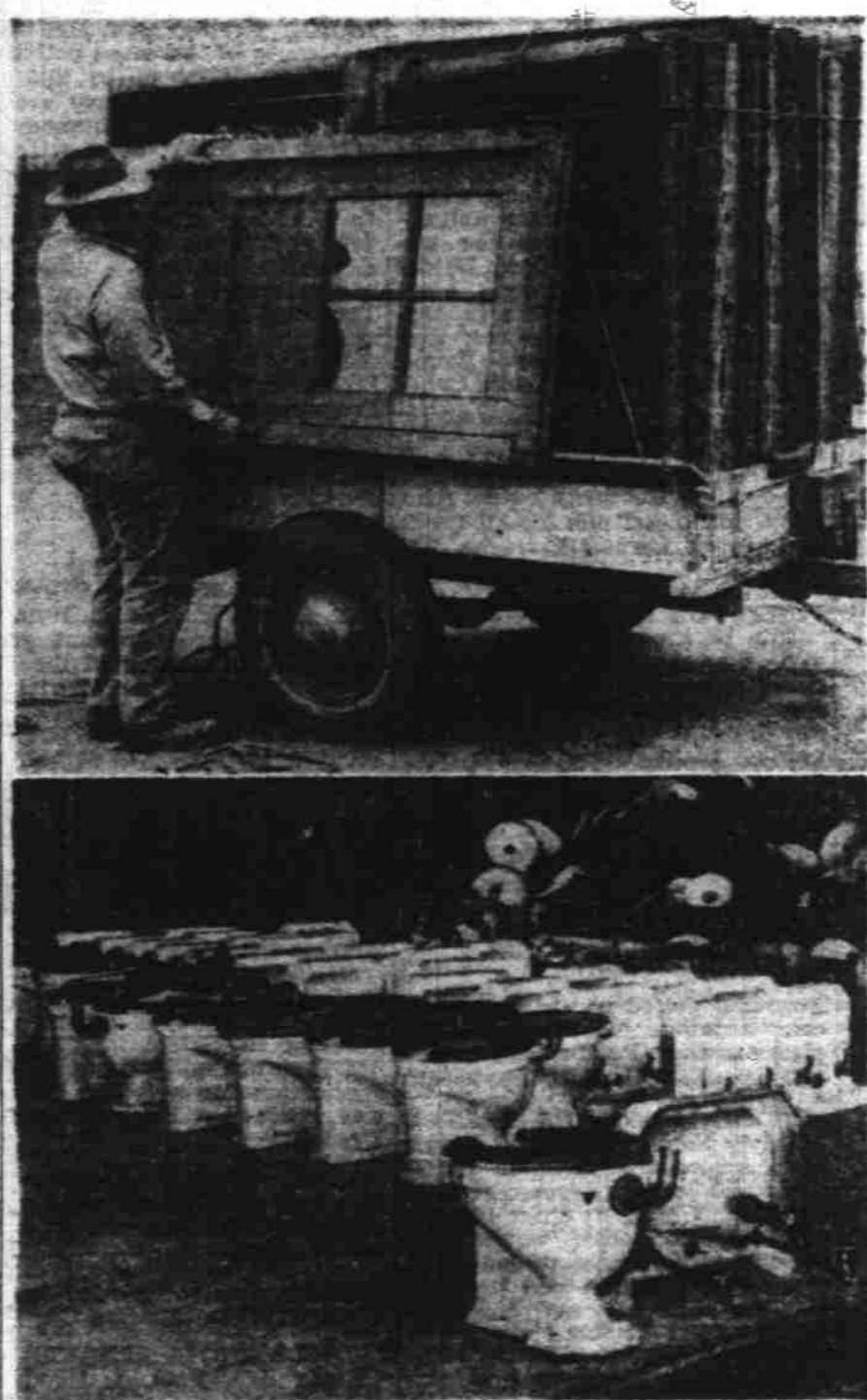
CAMP ADAIR, May 8.—Amateur home builders are solving their material problems with salvaged lumber, doors, windows and plumbing fixtures from Camp Adair. Four wrecking companies are busy tearing down the barracks, and buildings of the deserted camp from which come the toilets and wash bowls shown in lower picture. In the upper picture, Jim Booth, 970 Mth st., loads a door on his trailer along with windows and screens. (Photo by Don Dill, Statesman staff photographer.) (Story on Page 1).
