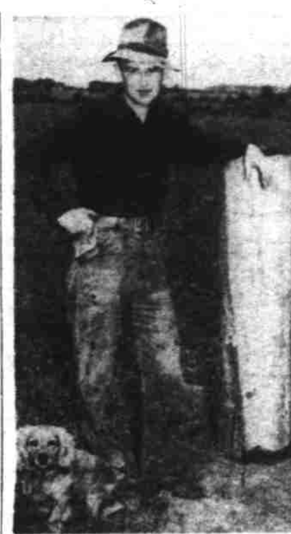
Bob Hamilton, progressive Polk county farmer, was caught in the act of resetting his fence. The iron posts, eight-feet long, are 13 years old. Four feet of the post go in the ground. The corner or anchor posts are of cedar, fully ten inches across and also planted four feet down to assure firmness. If you have any stock, a good fence is half the battle won, says Hamilton. (Statesman farm photo)
