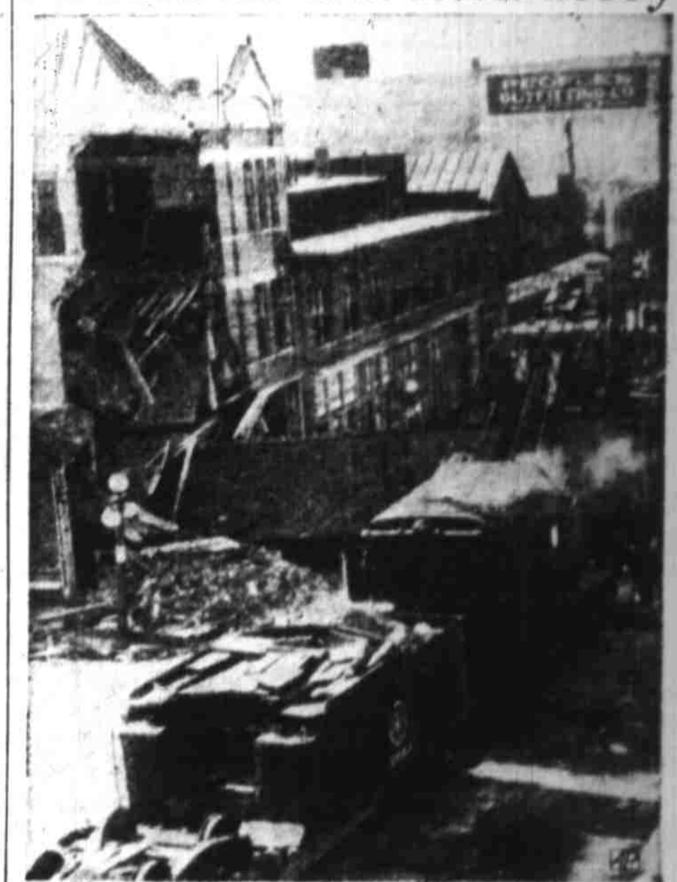
SPRINGFIELD, O., Oct. 14—A wrecking crane is busy extricating a refrigerator car that smashed into the lobby of the Frances hotel here today. It was one of three cars of a New York Central freight train derailed in the center of the city. (AP Wirephoto).
