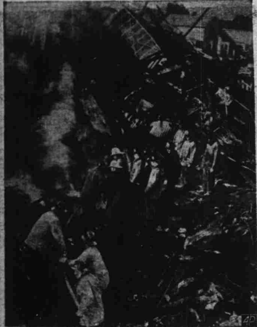
Firemen search for victims in the wreckage of a warehouse-apartment building destroyed by an unexplained blast at Santa Barbara, Calif. Five bodies were removed from the debris, while five other persons were injured. (AP Wirephoto)
