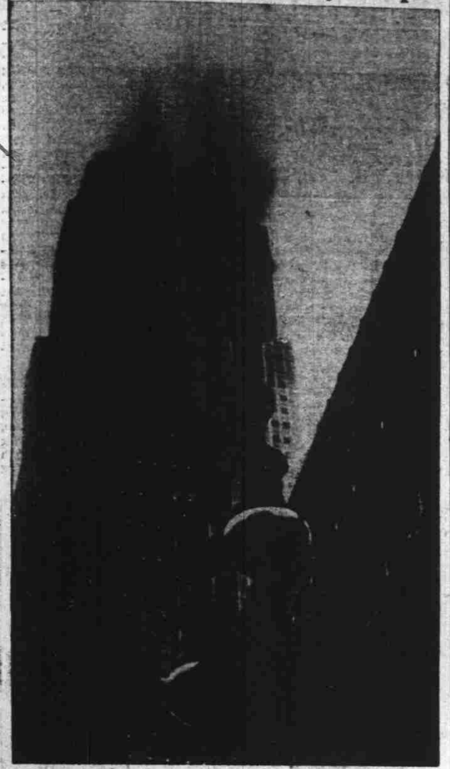
Smoke billows out from upper floors of the Empire State building Saturday morning after a plane crashed into the 78th floor of the structure. Fires were burning in 11 of the upper floors of the building. (AP Wirephoto). (Additional picture on page 2)
