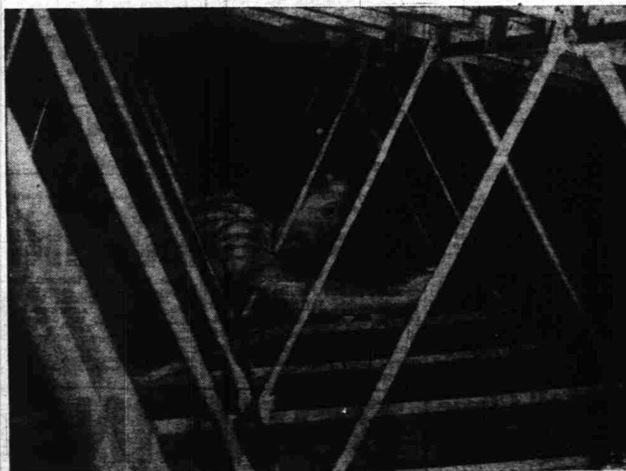
AIRPLANE SEAMSTRESS —Inside the wing of a big clipper plane at Pan American's base at LaGuardia Field, N. Y., Marion Randall of Flushing, L. I., sews on the fabric section of the wing of the 43-ton flying boat.
