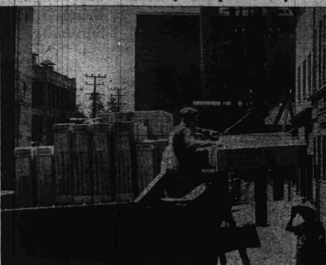
Loading packaged and sections of Quonset huts manufactured by Oregon Pulp & Paper Co. lumber division for use of the navy in the tropics, L. E. Bates and Robert Dennis guide the crane load which A. F. Solte, standing below, started on its way to them. The company ships a carload a day from this factory on Front street in Salem.
