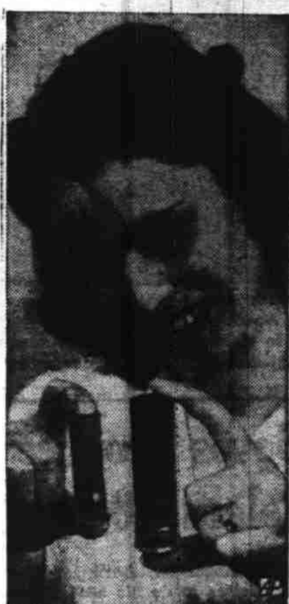
STARTER —Molly Keane compares an airplane starter shell (right), made at Winchester Repeating Arms Co. plant at New Haven, Conn., with an ordinary 12-gauge shotshell. Cartridge furnishes single powerful impulse starting airplane motor.
