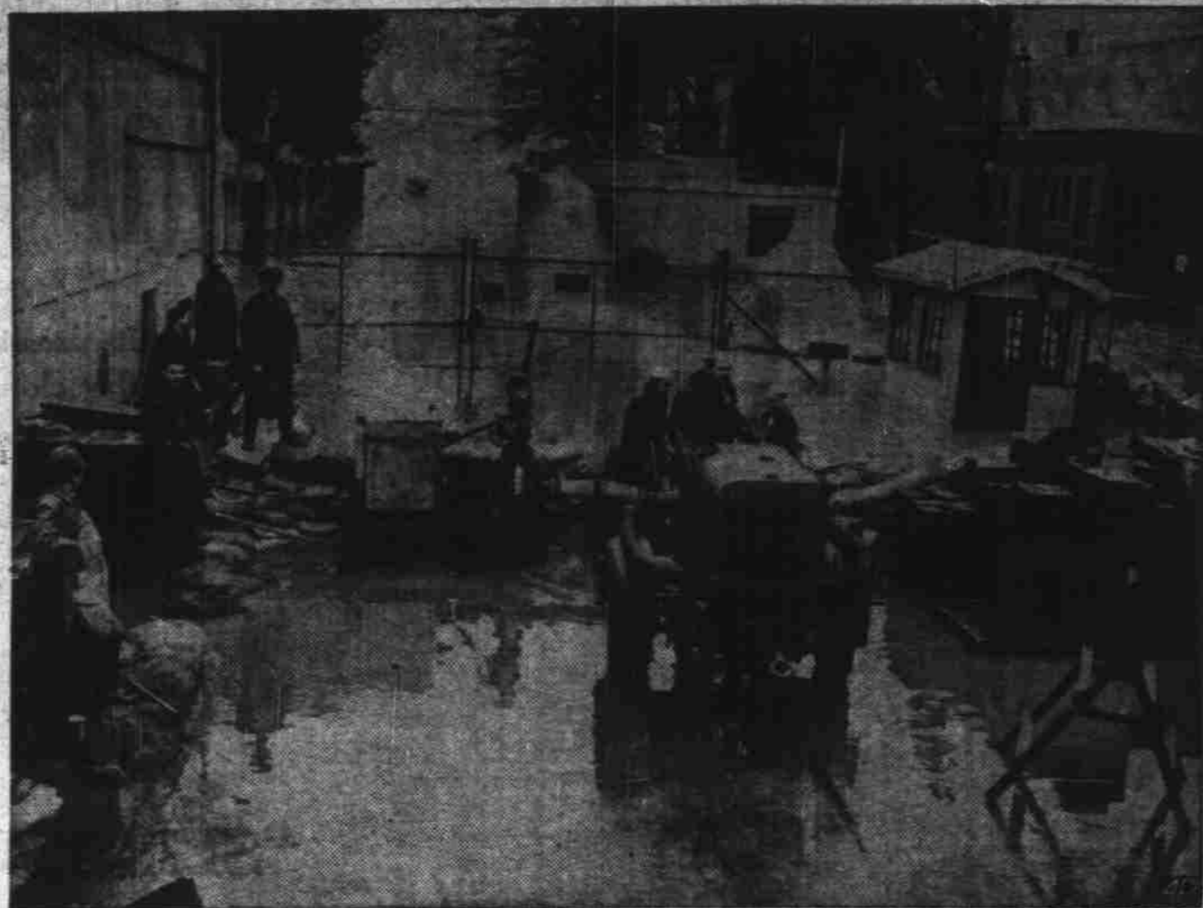
Three coast guardsmen operate an auxiliary pumper at the R. G. LeTourneau plant, Peoria, Ill., enabling continued work on war contracts. Sprays of water from the pump can be seen in the background. The rising flood of the Illinois river threatened several industrial units at Peoria. — Associated Press Telegram.
