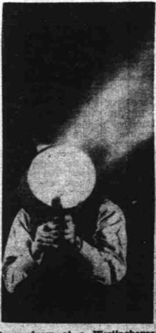
An engineer at a Westingho plant tests a new light gun that soon will be flashing signals to United Nations planes in war sones throughout the world. The pull of a trigger sends a 500,-000-candle power beam of light a mile into the air; another pull flashes a green or red stream of light. At airports whose radio transmitters are ellenced to preenemy, these light guns will 43 malt drin 45 loud clam 46 small fine fliers with powerful light gun ed. green and white lights.—
