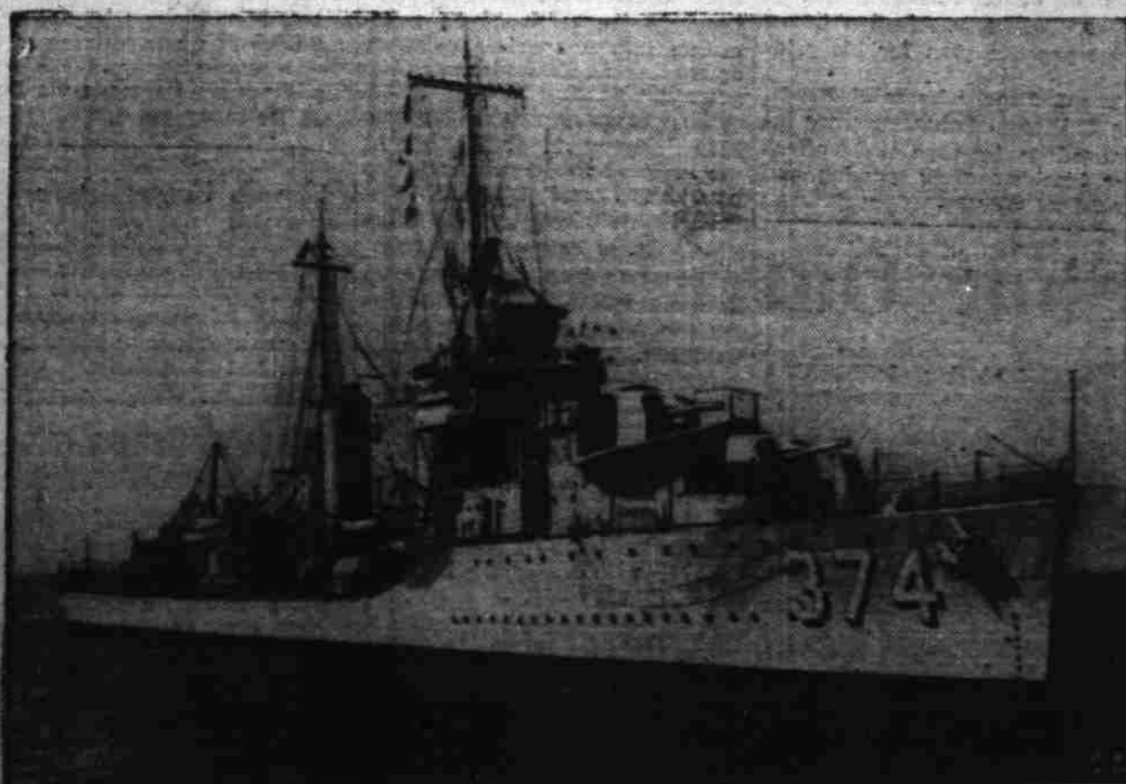
ONE OF UNCLE SAM'S DESTROYERS —The U.S.S. Tucker (above), a 1,500-ton destroyer completed March 29, 1927, has a speed of about 26 knots.
