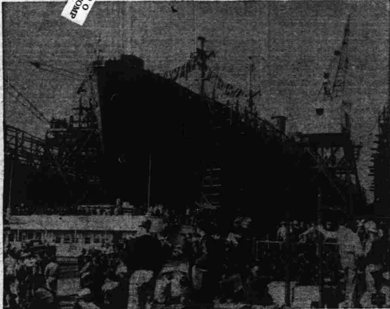
Ten days from keel-laying to launching, the 10,500-ton Liberty freighter Joseph N. Teal (above) hit the water in the shipyards of Henry J. Kaiser at Portland. This picture was made during the launching ceremonies. The amazing speed record cut 14 days off the best previous record for shipbuilding. The yard intends to have the boat ready for the sea Sunday and if it succeeds will have delivered a major cargo vessel in two weeks.—Associated Press Teletext.
