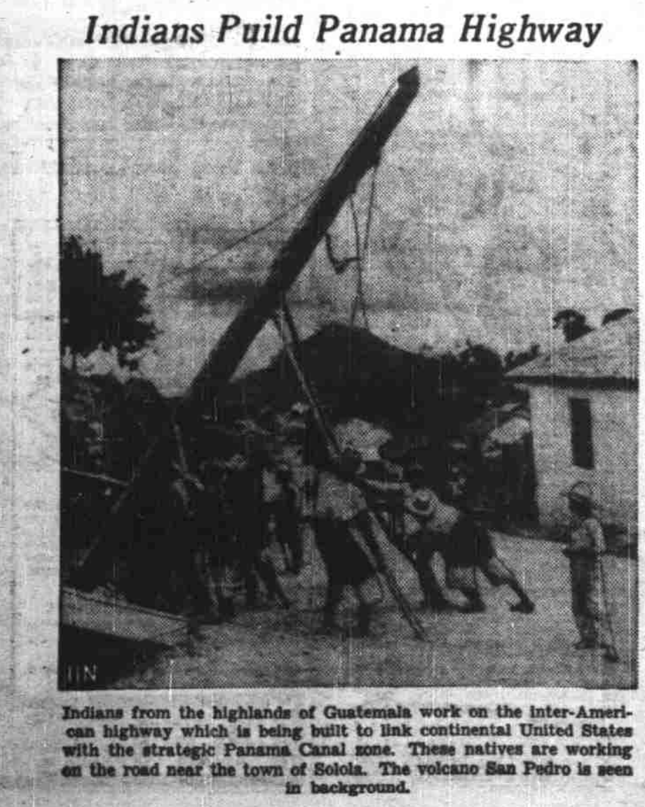
Indians from the highlands of Guatemala work on the Inter-American highway which is being built to link continental United States with the strategic Panama Canal zone. These natives are working on the road near the town of Solola. The volcano San Pedro is seen in background.
