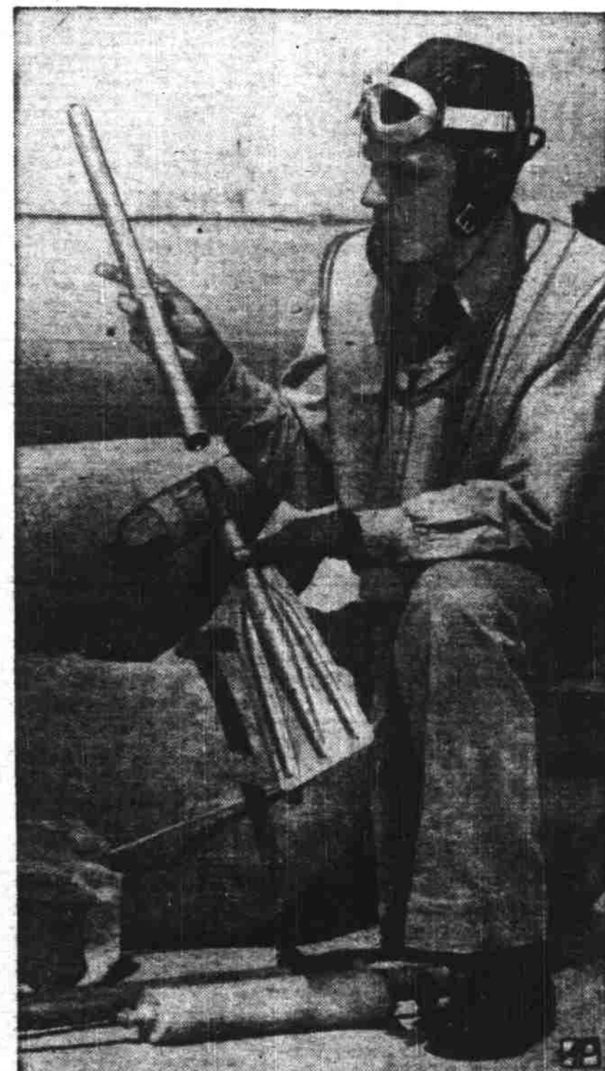
AN OAR IN A PINCH —Aviation Chief Machinist's Mate Harold F. Dixon exhibits one of the two-piece collapsible oars which are part of the self-inflating life raft equipment carried by aviators operating over long stretches of water. Other equipment in the raft includes a pump, signaling mirror, balling pouch, whistle and cord.
