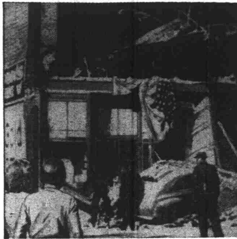
Nope, you're wrong, this is not a war picture. And the damage pictured is not from an enemy bombing raid. A taxicab went berserk in Vincennes, Ind., smashed into the building and caused all this damage. The driver, luckily, escaped serious injury.
