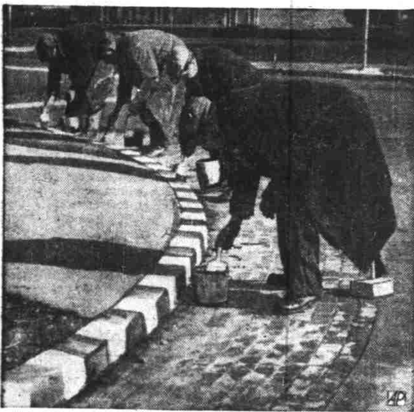
BLACK AND WHITE —Getting ready for blackouts—rehearsals and the real thing—Philadelphia workmen daub white paint on the curbing of a street, in a striped effect that will make the curbs visible to motorists and pedestrians.
