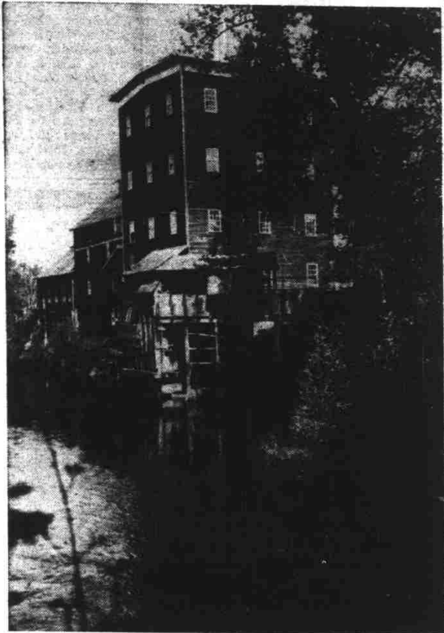
This old mill, while in a picturesque setting, is considered a fire hazard and now that Silverton owns the property it will be torn down.
