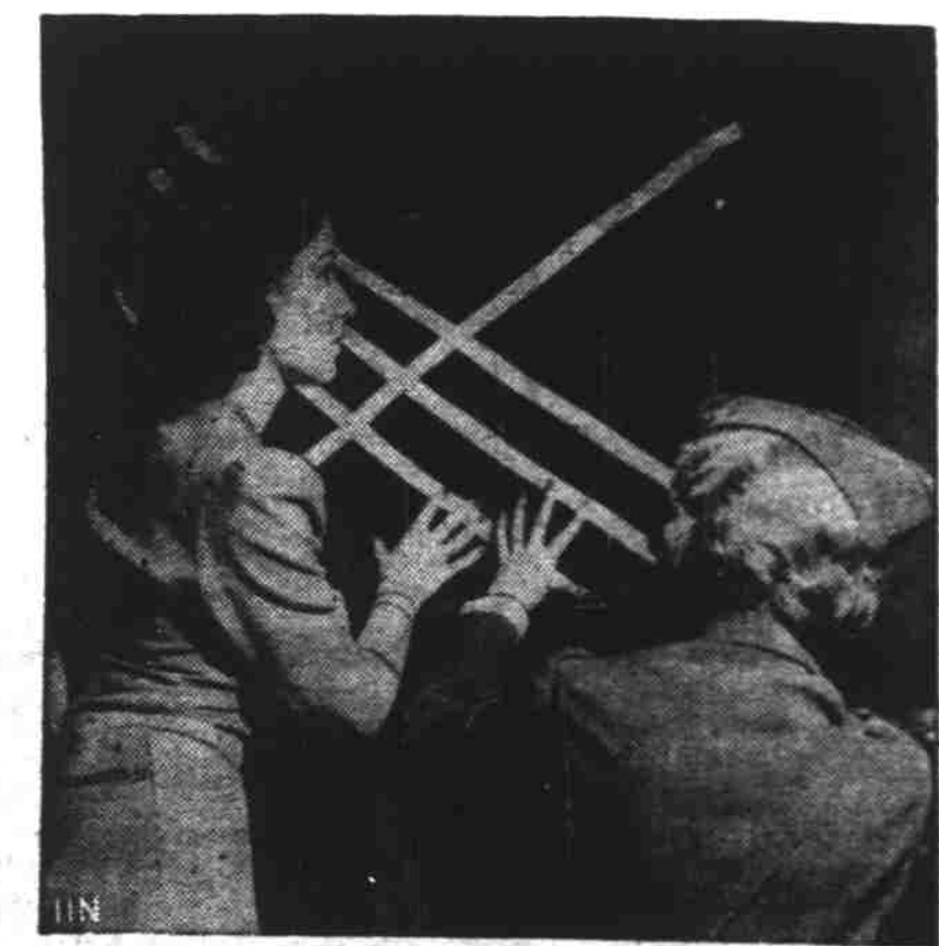
Preparing for possible enemy air attack, New Yorkers are looking to their home defense, including precautionary measures against building destruction. Here a housewife and an instructor of the American Women's Volunteer Service tape up a window to prevent wounds from flying shrapnel of glass should an air raid come.
