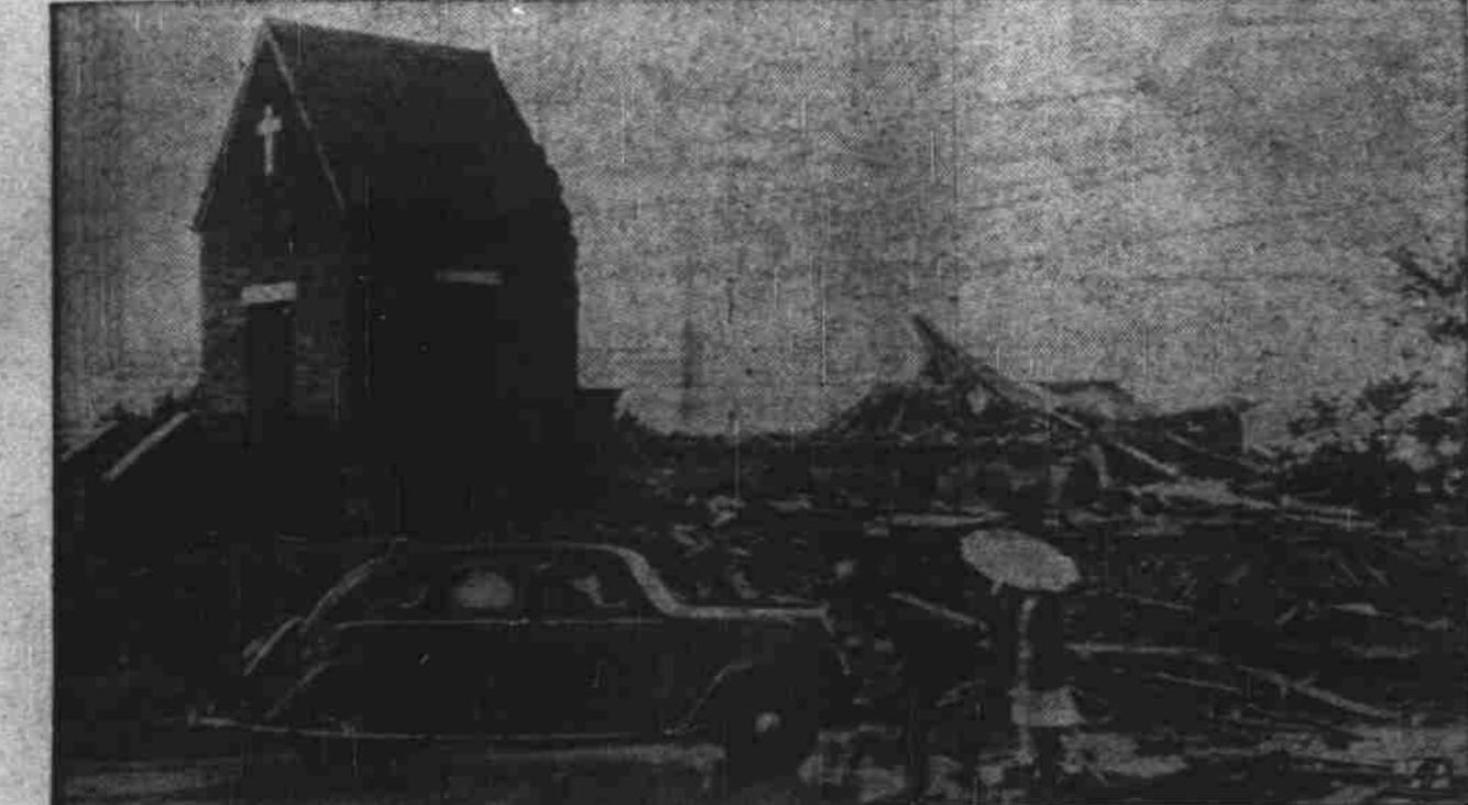
A tornado wind sliced away all but the front section of the New Arlington Methodist church on the eastern edge of Kansas City as it followed an erratic course, killing a woman and child, injuring a dozen persons and causing heavy property damage.
