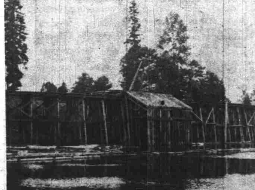
Typical of the many log dumps along the Willamette is this big one (above) operated by the Molalla Logging company near Canby and designed to handle 600,000 feet a day. Twenty-eight company-owned trucks and 20 contract units making hauls averaging 30 miles use its facilities.
