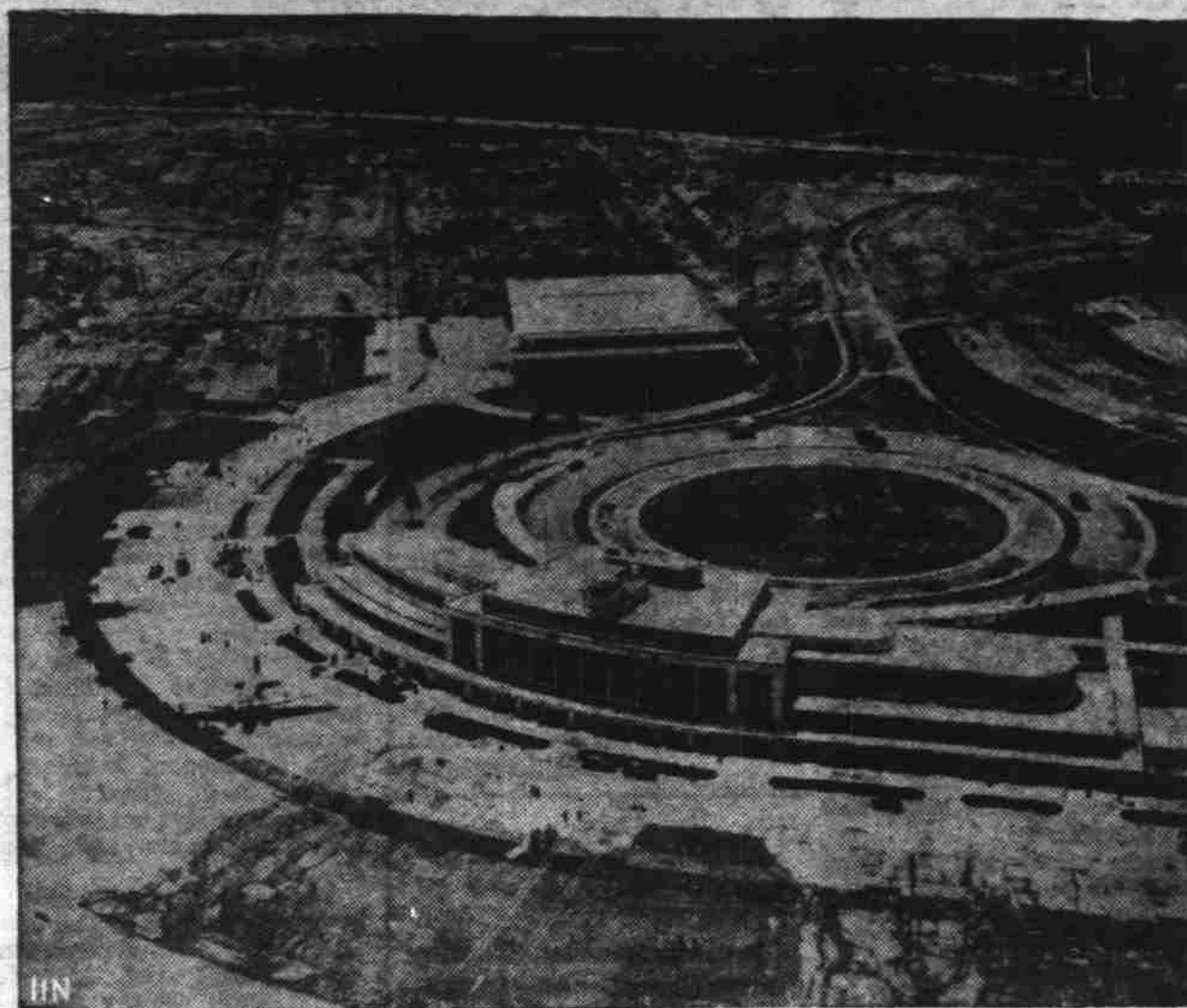
Washington's National airport, which cost $15,000,000 to build, has been officially opened for traffic. Large waiting rooms, dining rooms and a promenade deck to watch the arrival of planes are features of the new port. One room has been designated "President's Room" and will be used to receive distinguished visitors.
