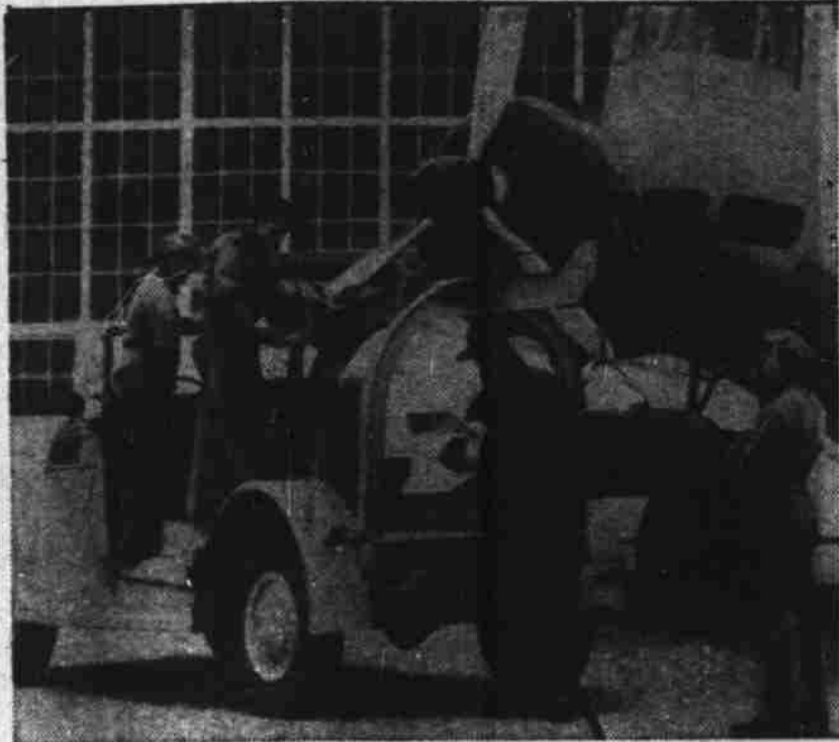
A familiar piece of motorized equipment around US army air corps bases these days is this new bomb service truck, shown being demonstrated near a giant US army bomber. Manufactured by the Ford Motor company, the special trucks are rigged with derrick and windlass to facilitate handling of bombs weighing from 600 to 1200 pounds. These trucks are used for towing bomb trailers or carrying bombs such as the 600-pounder shown above, from storage points to the airplane.
