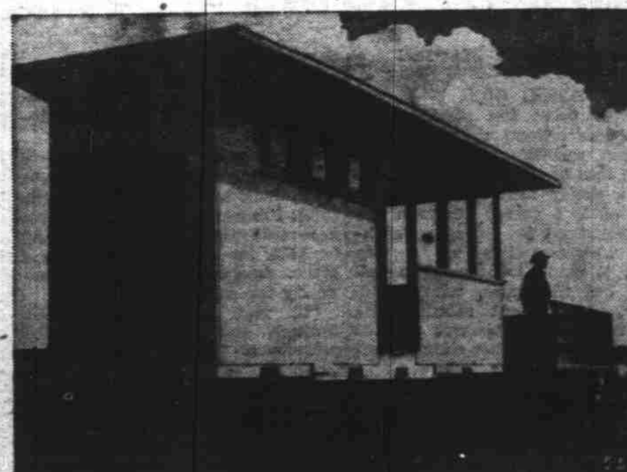
HOMES BY THE PIECE —To supply a demand for workers' homes, TVA is moving small, factory-built cottages in sections, like the one shown, to dam sites in the Tennessee valley. This section is headed for Pickwick dam home colony.
