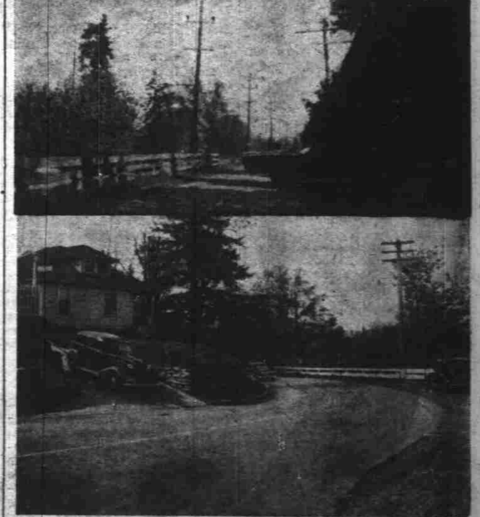
Here are two of the hazards that South River road improvement proponents hope to see eliminated: Top, delivery truck parked by necessity, on the narrow road at the Schindler dairy, which lies within the city limits; below, sharp, blind curve where road enters Hillier street, with steep driveway entering from apartments on the knoll above. It is proposed to extend the road northward to enter at Owens street in a broad, clear-vision curve, and to widen the roadway to the south, which has a right of way only 27 feet in width. Part of the original right of way was sold to the Oregon Electric railway years ago.
