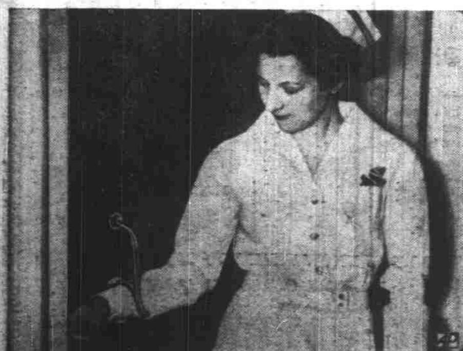
WHEN HANDS ARE FULL —Mildred Albritton, chief dietitian at Fitzsimons hospital, demonstrates how doors in the new hospital building can be opened by a nurse who has both hands full, leaving or entering the room. A wrist will serve.
