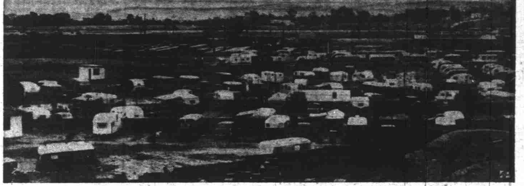
ROOMS ON, AND WE DON'T MEAN CANNON—California, like other states where defense activity is rushing, has a building boom on its hands, especially in those sections where quarters for the soldiers are being constructed. Here are scenes from San Diego; additional naval facilities and a coast artillery corps replacement center to house 8,500 men are being built there. In upper view is the barracks being built at Camp Cassan near San Diego. Below is a trailer colony for workmen unable to find homes.
