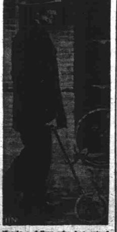
Here's a fellow who has solved the problem of wandering in blacked-out cities in Europe by developing a wheeled came with a spetlight which focuses on the ground a few feet in front of the pedestrien. The power is by bat-teries attached to the case. The pisture was taken in Amsterdam, Molland.
