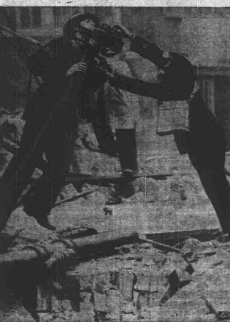
A British censor approved caption says this picture was made just 30 seconds after a bomb exploded in a London street. The two bobbies are sniffing a lamp post to determine if the bomb blast has caused a gas leak which might result in a fire or another explosion.
