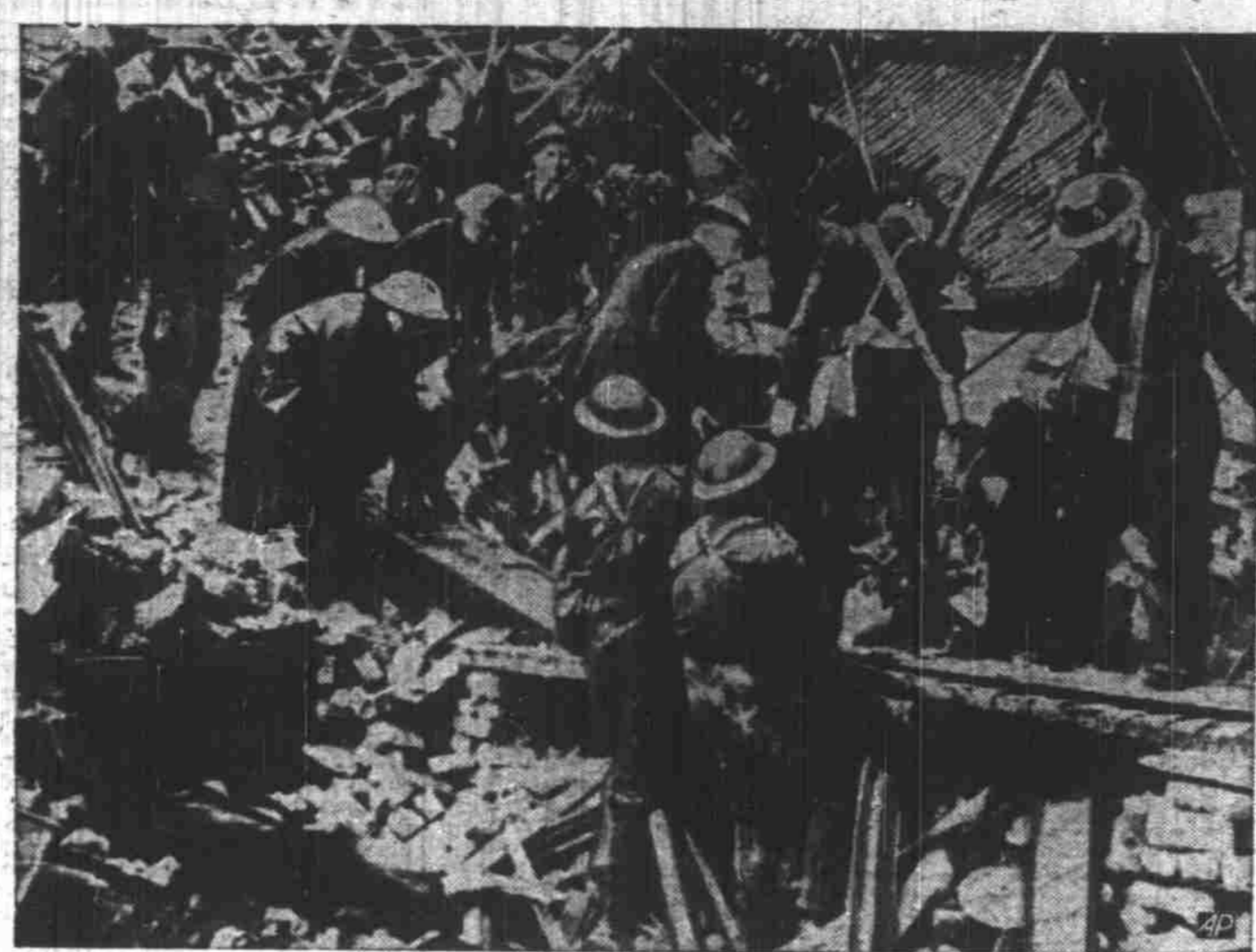
Out of the ruins of a London building wrecked in a German air raid, British rescue workers bring one of the persons wounded in a bomb blast. British sources said some of the persons injured in this structure were trapped for seven hours before being rescued. This picture was cabled from London to New York.
