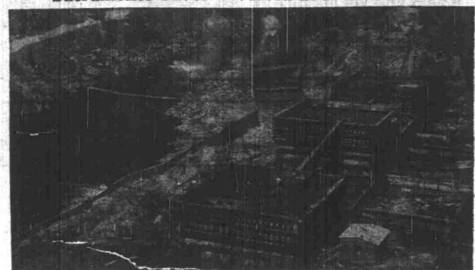
Initial opening in a dike at upstream end of a newly prepared canal was dynamited recently to divert the course of the Sacramento river to make room for work at California's huge Shasta dam, near Redding. Note men in foreground hiding behind one of the big concrete blocks comprising part of the dam, as the blast is shot at intake of the temporary man-made channel.--IIN photo.
