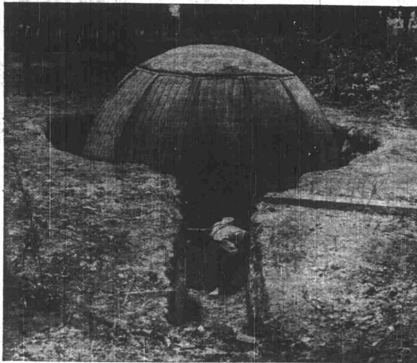
BITTER PILL—FOR AN ENEMY —At least one "John Fublie" inspects first-hand a bomb-resisting pillbox demonstrated to army and navy leaders in Washington at an isolated spot along the Potomac. Built of concrete in five hours, complete with gun openings and trench approach, the pillbox supported weight of three men a few hours later.
