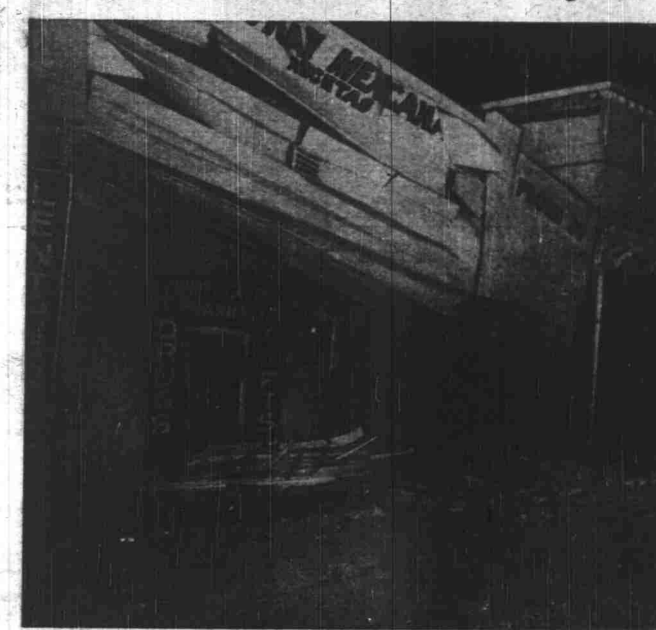
Samples of the terrific havoc resulting from the earthquake which hit the Imperial valley on Saturday night. Top photo shows wreckage of a drug store; lower photo shows two automobiles after collision from a building had fallen on them. Both are scenes in Brawley.—IIN photos.
