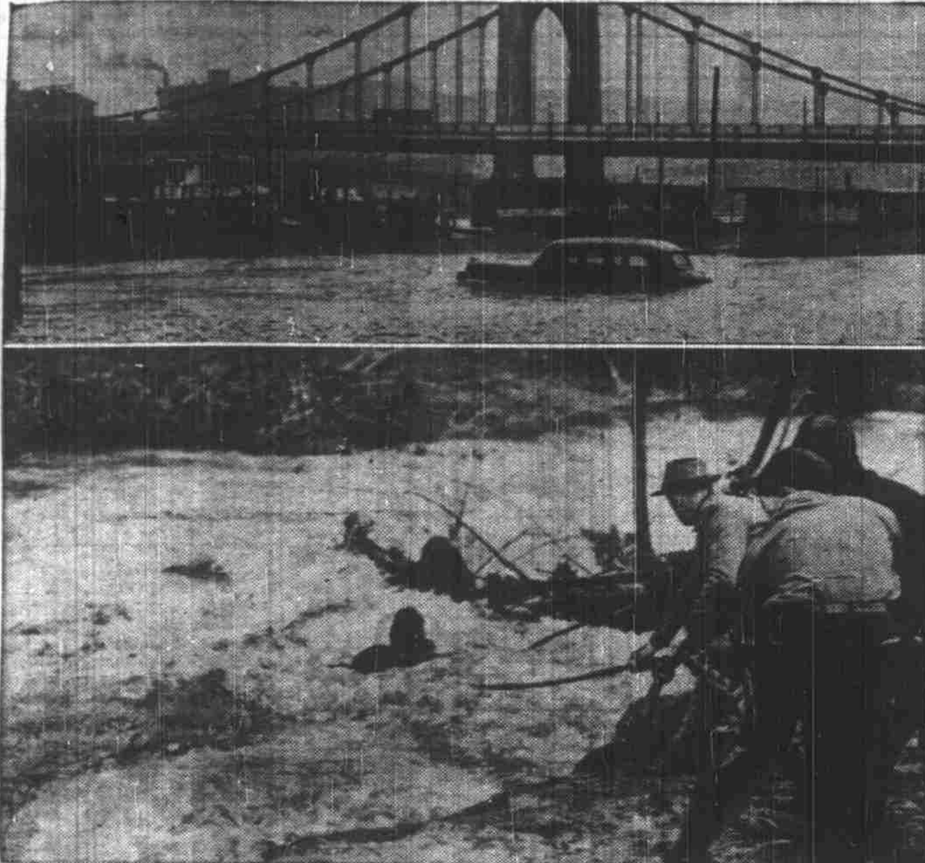
Flood scenes around Pittsburgh, Pa., as the Allegheny river reaches flood levels following eastern torrential rains. Top picture shows a stranded automobile on Pittsburgh's low-lying flooded north side. Bottom, a Pennsylvania highway foreman being rescued from raging Robinson Run, near Pittsburgh, after he had fallen in while checking flood level heights.—H.N. photo.
