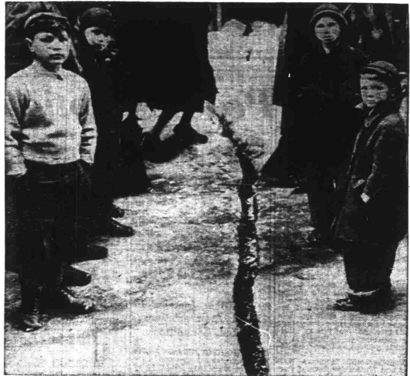
A group of wide-eyed Shenandoah, Pa., school children gather about a crevice in the earth, one of the cracks which caused a six-block segment of the city, built over an abandoned anthracite mine, to sink slowly into the mine workings. There was no loss of life or injury.—H.N. photo.
