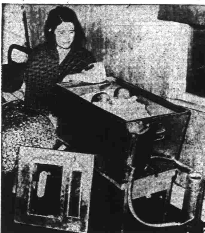
This kerosene burning portable incubator, costing $50, is undergoing tests in Maryland's fight against high death rate among county babies born prematurely. Mrs. Irma Griffin, of Salisbury, finds it also works well as a crib for her twins.
