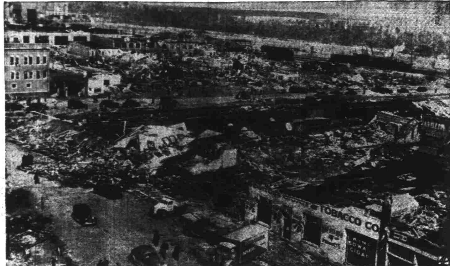
Only two or three buildings were left standing in this section of Albany, Ga., after a tornado struck. Homes and business houses were splintered and boxcars overturned like toys. At least 17 persons were killed and 300 injured. Damage was estimated at $5,000,000.
