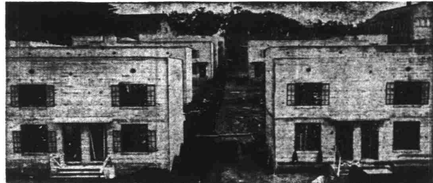
Nearly 60 per cent complete is the US Housing authority's low rental housing unit being constructed in San Francisco. Model for other coast construction to follow. One hundred eighteen families are expected to occupy the group about June 1. Partially finished part of the construction, called Molly Circle, is shown above. All utilities will be included with rental totaling about $4 a room. The project is first in the nation west of the Rockies.
