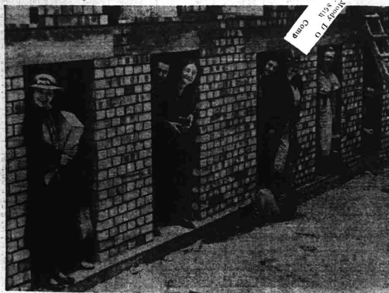
London has as yet been free of enemy air raids, but an elaborate system of bomb shelters and air raid alarms continues to be pushed to completion by the British government. Pictured above is a group of housewives in southeastern London at entrance to a line of novel brick and concrete bomb shelters. Each compartment is shelter for a single family and, according to reports, makes a comfortable sitting room. (HIN photo.)
