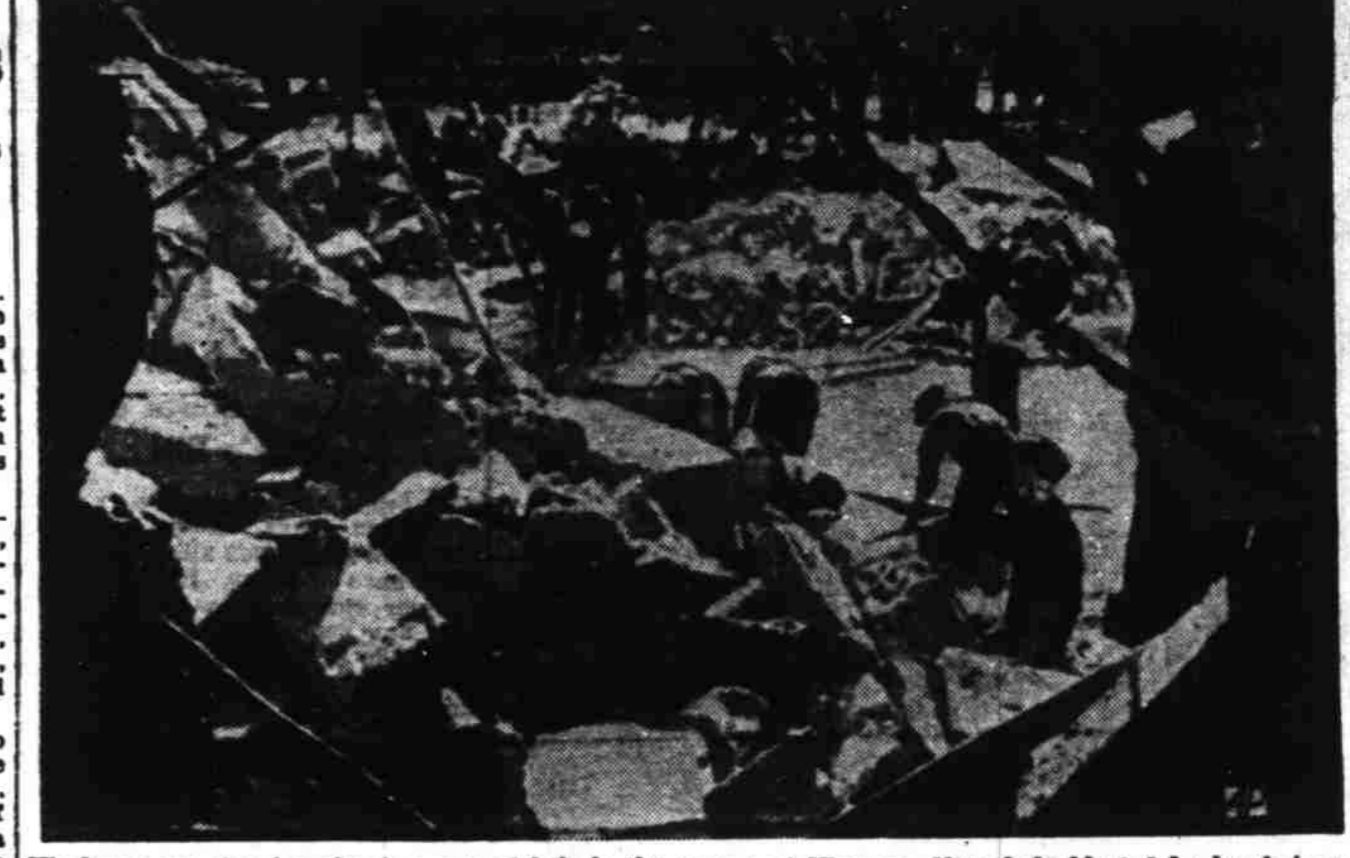
Workmen are showing clearing away debris in the center of Warsaw. Note hole blasted by bomb in a wall.
