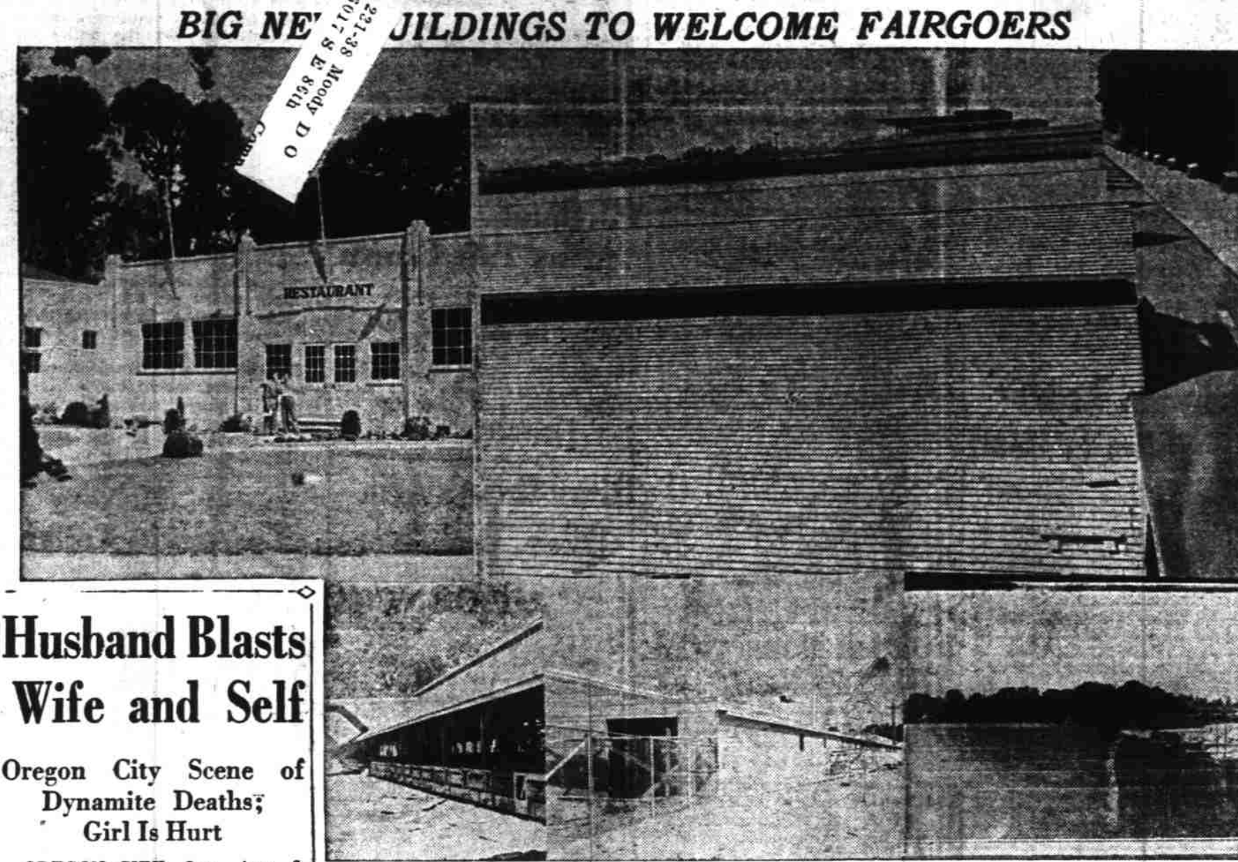
Both expanse and attractiveness of new state fair buildings being completed this summer are illustrated above. New restaurant-auditorium building, upper right, with J. D. Mickle, director of agriculture, and Leo Spitzbart, fair manager. Upper and lower right photos indicate immensity of new livestock pavilion, which is 722 feet long and 240 feet wide and will house 5000 animals.
