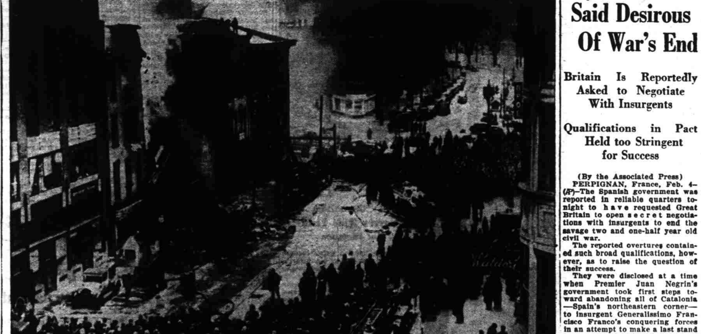
After 26 hours of digging in smoke-blackened ruins, searchers late Saturday found bodies of some of the eight firemen killed Friday when a five-story building in Syracuse, N.Y., collapsed while they were fighting a fire on the third floor. This picture was snapped just as the front wall collapsed into the street.—AP Telemat.
