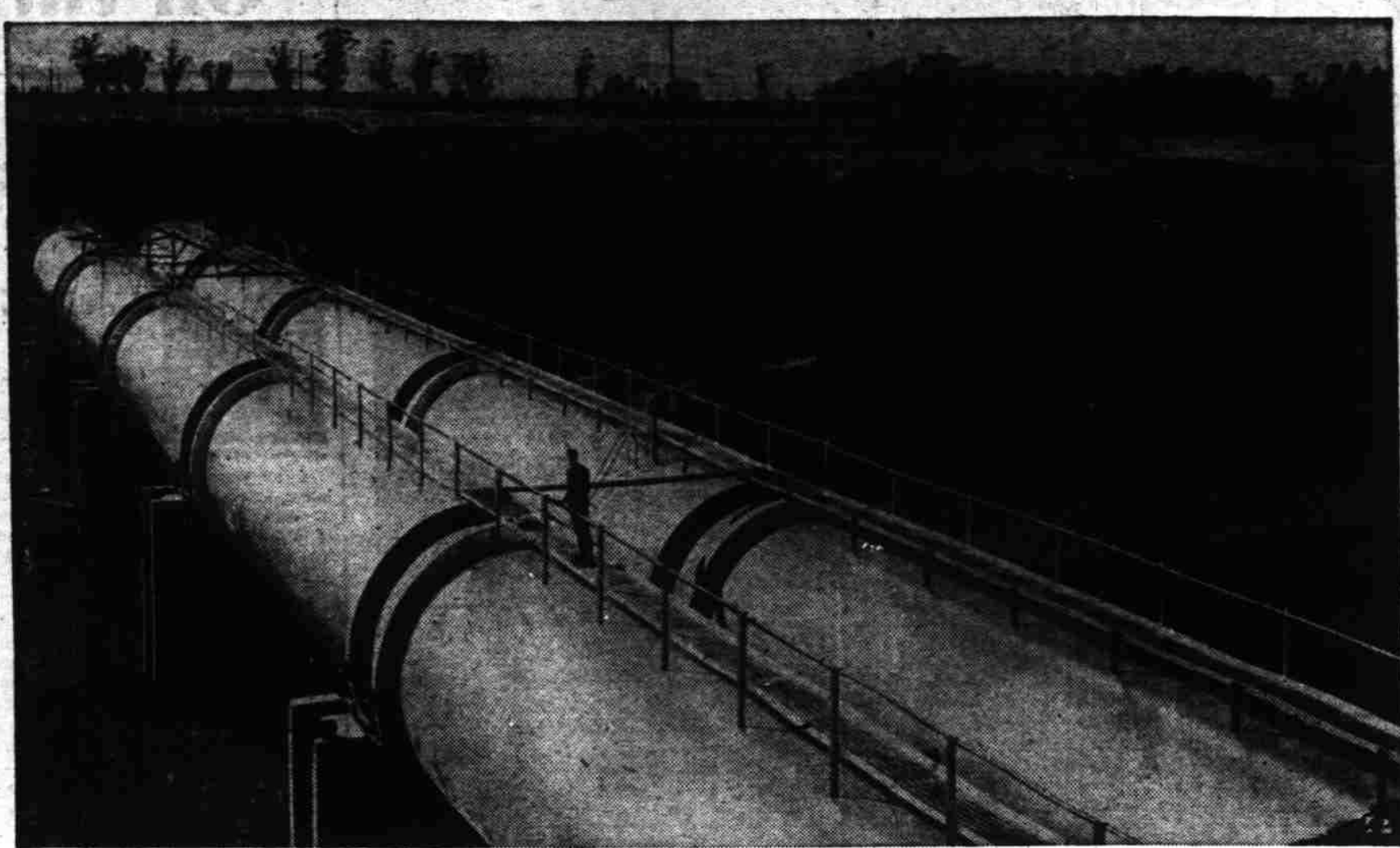
WATER FLOWS UNDER WATER at this point of the All-American canal one mile west of Calexico, Cal., for above two lines, each composed of five sections of 15 1/2-foot diameter pipe, siphon canal water across the New River. Canal nearly completion.
