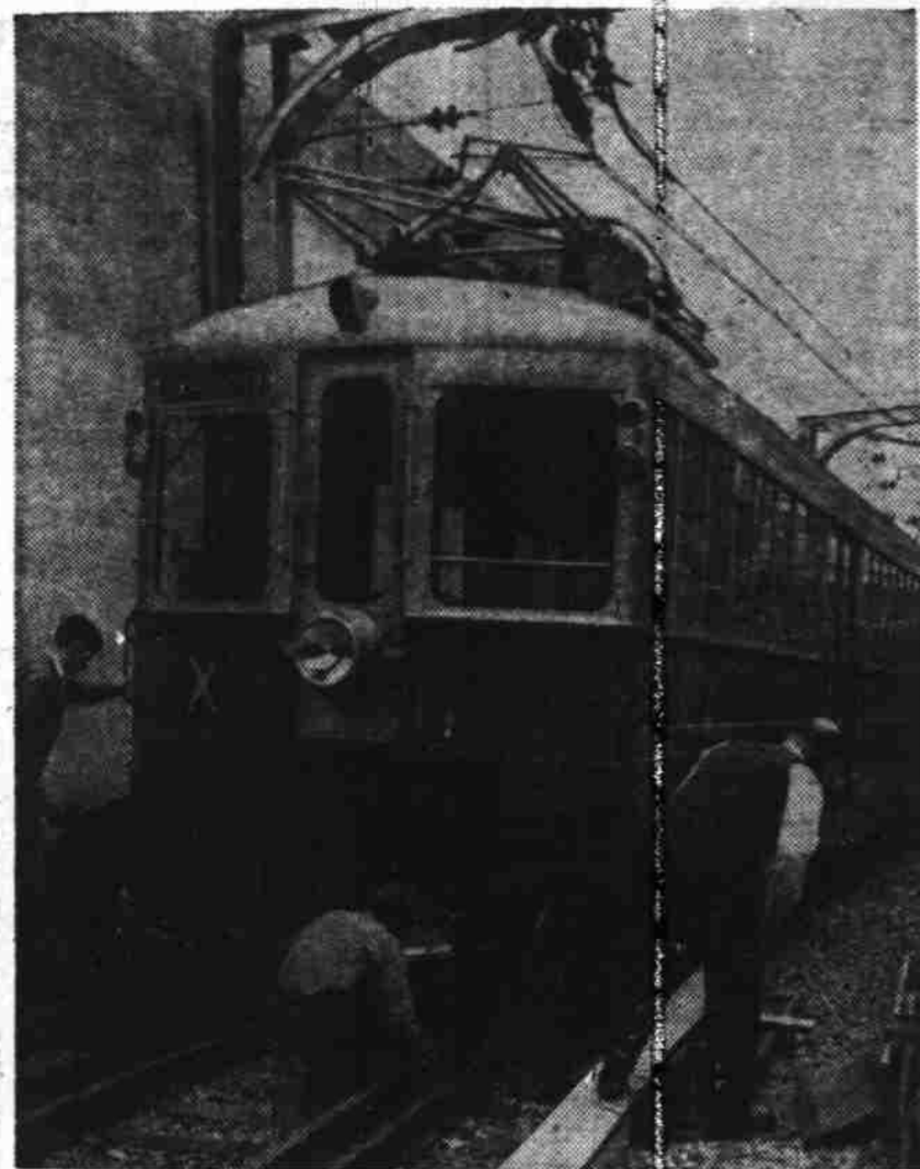
Gliding triumphantly over the San Francisco-Oakland Bay bridge, the first of the new streamlined interurban trains recently began a new era in transportation between San Francisco and East Bay cities. The inaugural trip, however, was somewhat humbled when the train reached the terminal. The power was not turned on. Photo shows several workmen pushing the train into the terminal station on the San Francisco side.—(HX).
