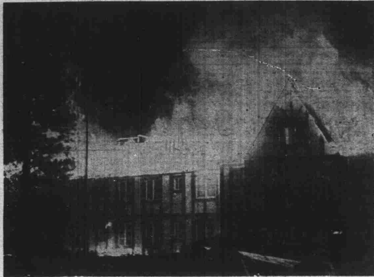
Arrowhead Lodge, palatial hostelry at Lake Arrowhead, Cal., is pictured as it was recently almost completely destroyed by fire. The blaze broke out in the kitchen. Loss was estimated at $500,000. Mountain fire fighting crews and CCC enrollees kept the flames from spreading to nearby mountain homes and forest land.—HN photo.
