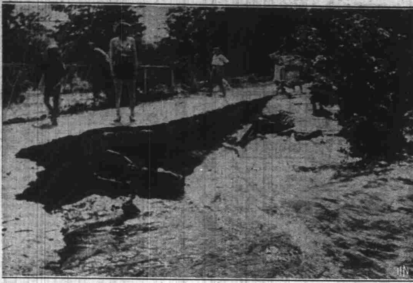
Part of this bridge has been washed away by seething flood waters at Debruce, N. Y., as successive days of rain drenched the East coast. Flooded conditions marooned motorists and campers, washed away bridges and closed parts of a railroad and state highway.
