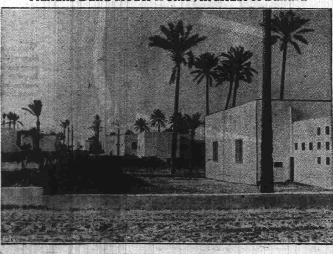
While the New Deal proceeds with housing projects on a vast scale, similar advances are being made in Africa where solid 14-inch thick cement houses are being built for Italian working men and their families at low rentals. Each home comprises a four-room apartment plus tiled kitchen and bath with ample garden space reclaimed and irrigated from the desert.
