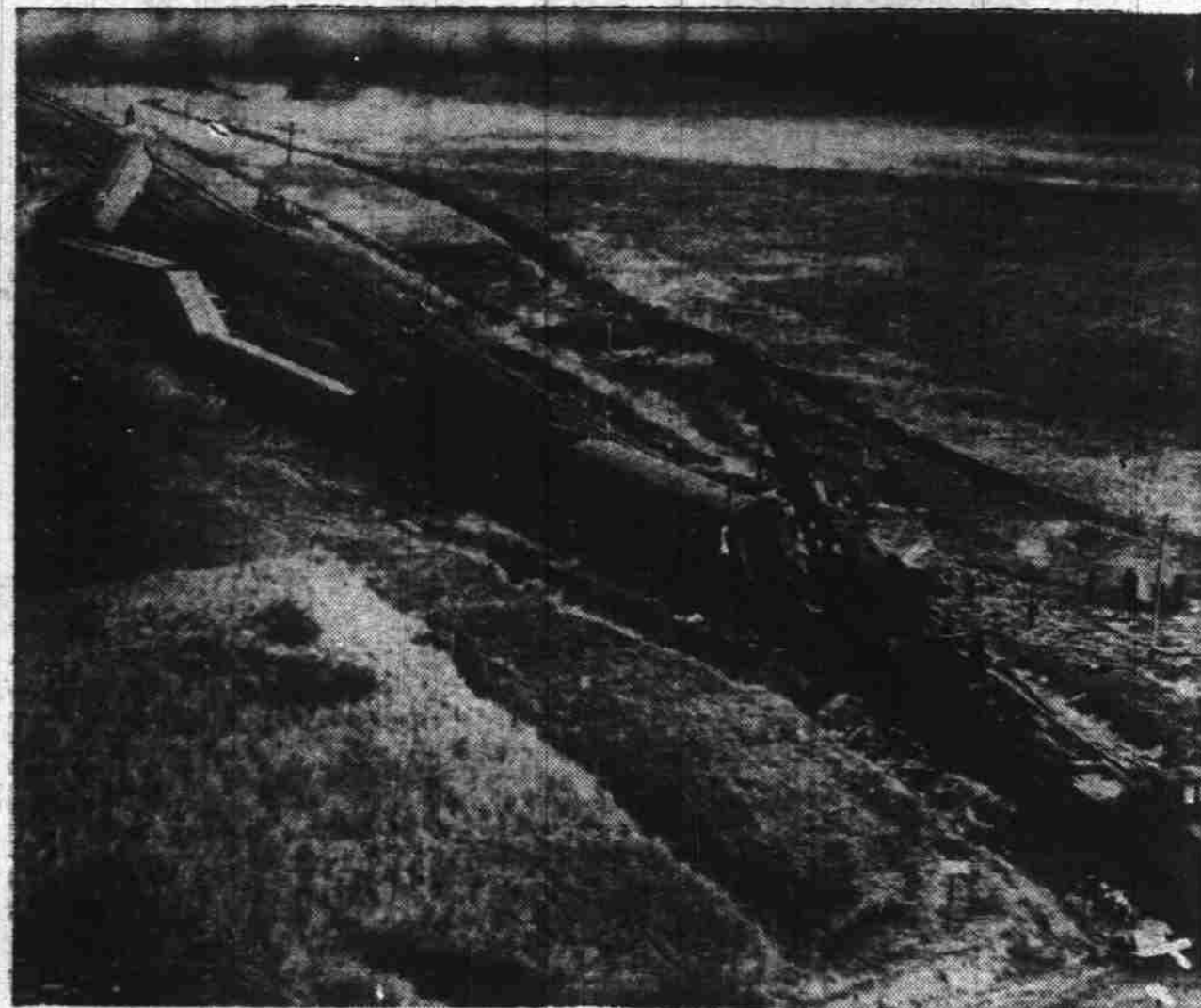
Six persons were injured recently when the Golden State Limited of the Rock Island line overturned near Trenton, Mo. The crack flyer was bound for Chicago from Los Angeles when it was derailed. Officials of the line blamed a broken rail for the wreck. Photo shows a wrecking car righting the coaches and setting them back on the tracks.—LIN photo.
