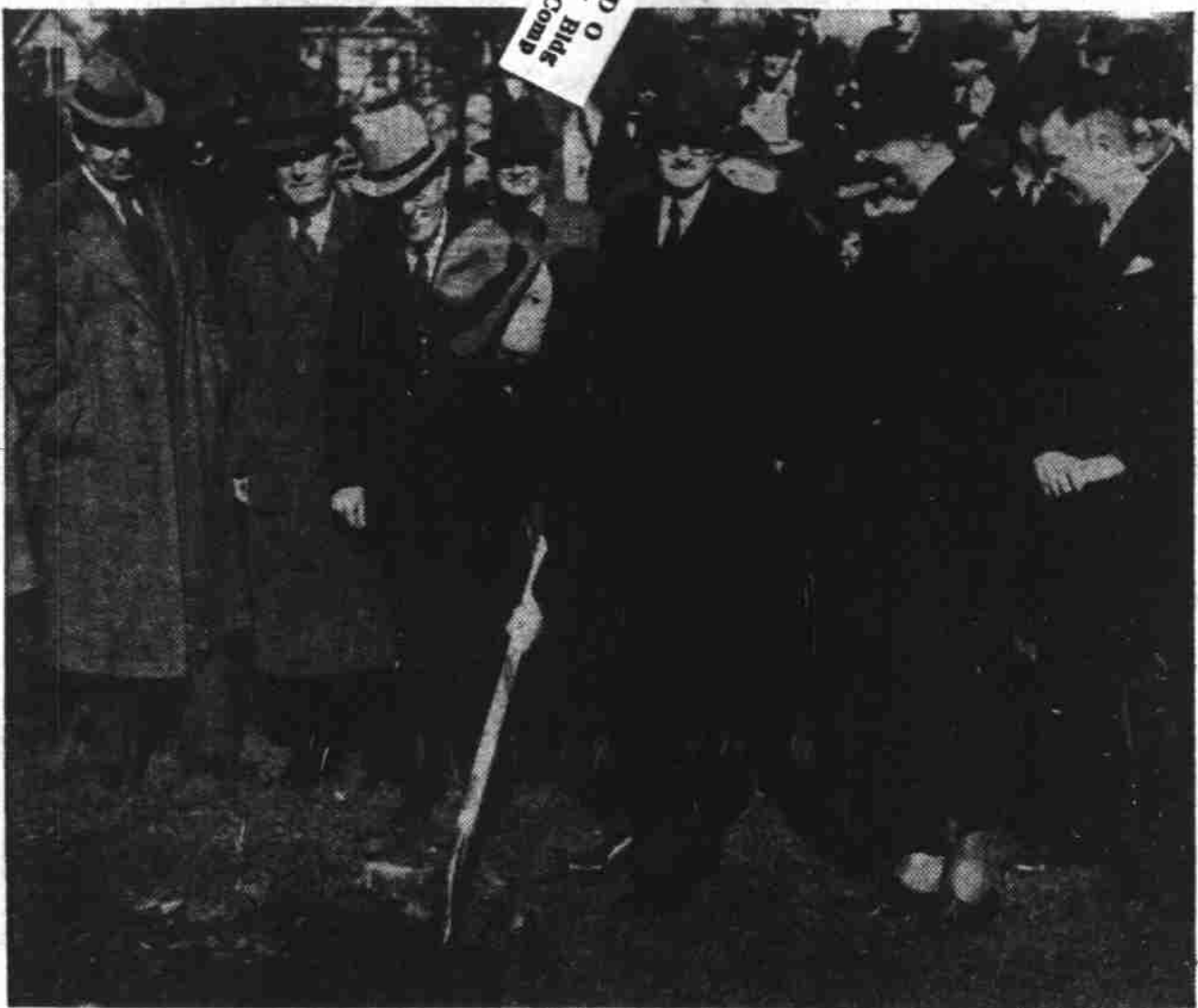
Governor Charles H. Martin turns the first spade of earth for the new state library-office building as other state officials, members of the capitol reconstruction commission and members of the library board look on.—Cut courtesy The Oregonian.
