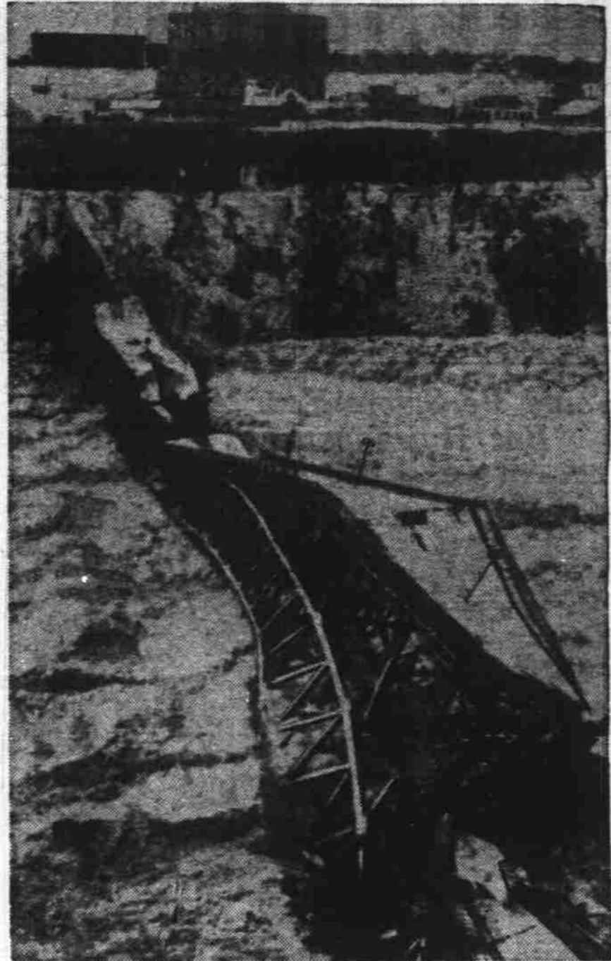
At the worst ice jam recorded in Niagara's history, the Falls View bridge, favorite honeymoon span, is pictured as it plugged into the deep gorge, a twisted mass of wreckage. The bridge had withstood the pressure of massive ice cakes piled 100 feet high for 48 hours. A crew of 12 men climbed to safety only a few minutes before the structure collapsed. A short distance below the falls, rising water and ice was reported to have seriously damaged a $25,000,000 power plant. The bridge spanned Niagara gorge dividing the United States from Canada.—IIN photo.
